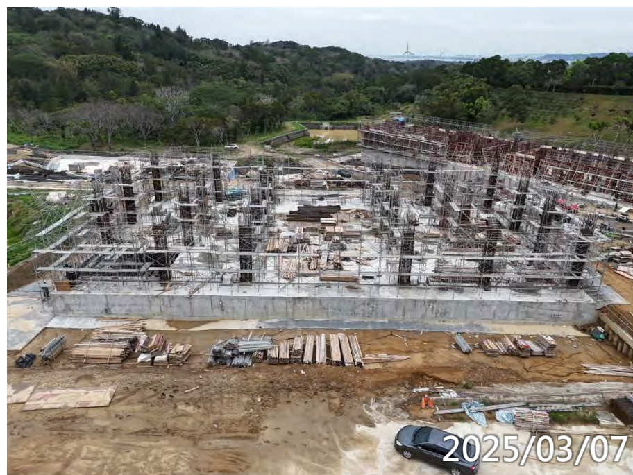
1F柱筋綁紮
