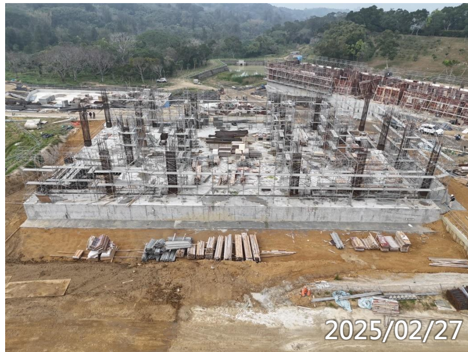
1F柱筋綁紮、土方回填
